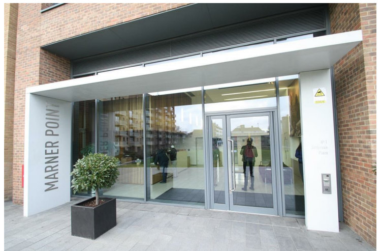
MARNER POINT ENTRANCE
