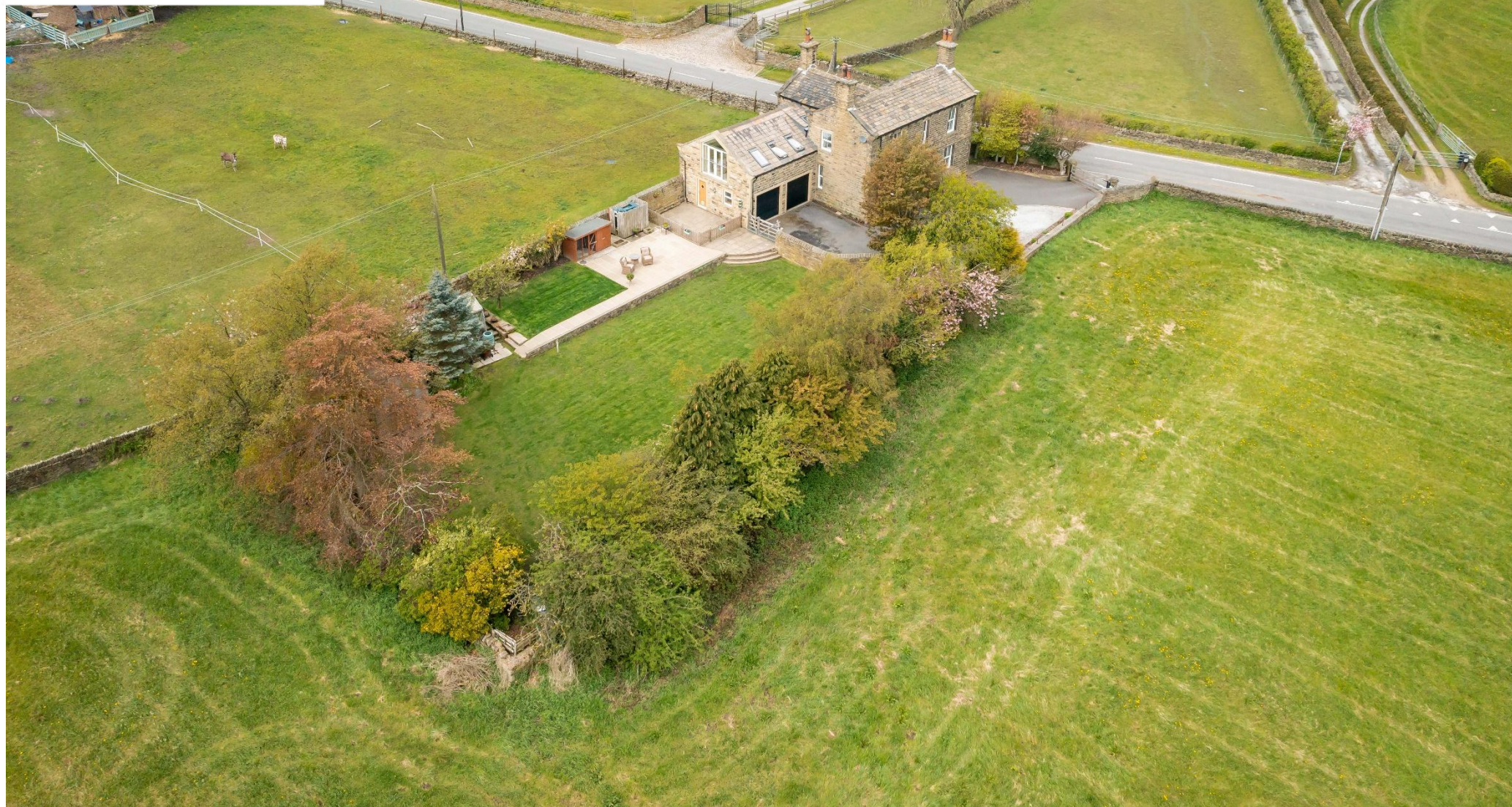
MARSHLANDS HOUSE AND ADJACENT BUILDING PLOT, MARSH LANE, SHEPLEY, HD8 8AY
