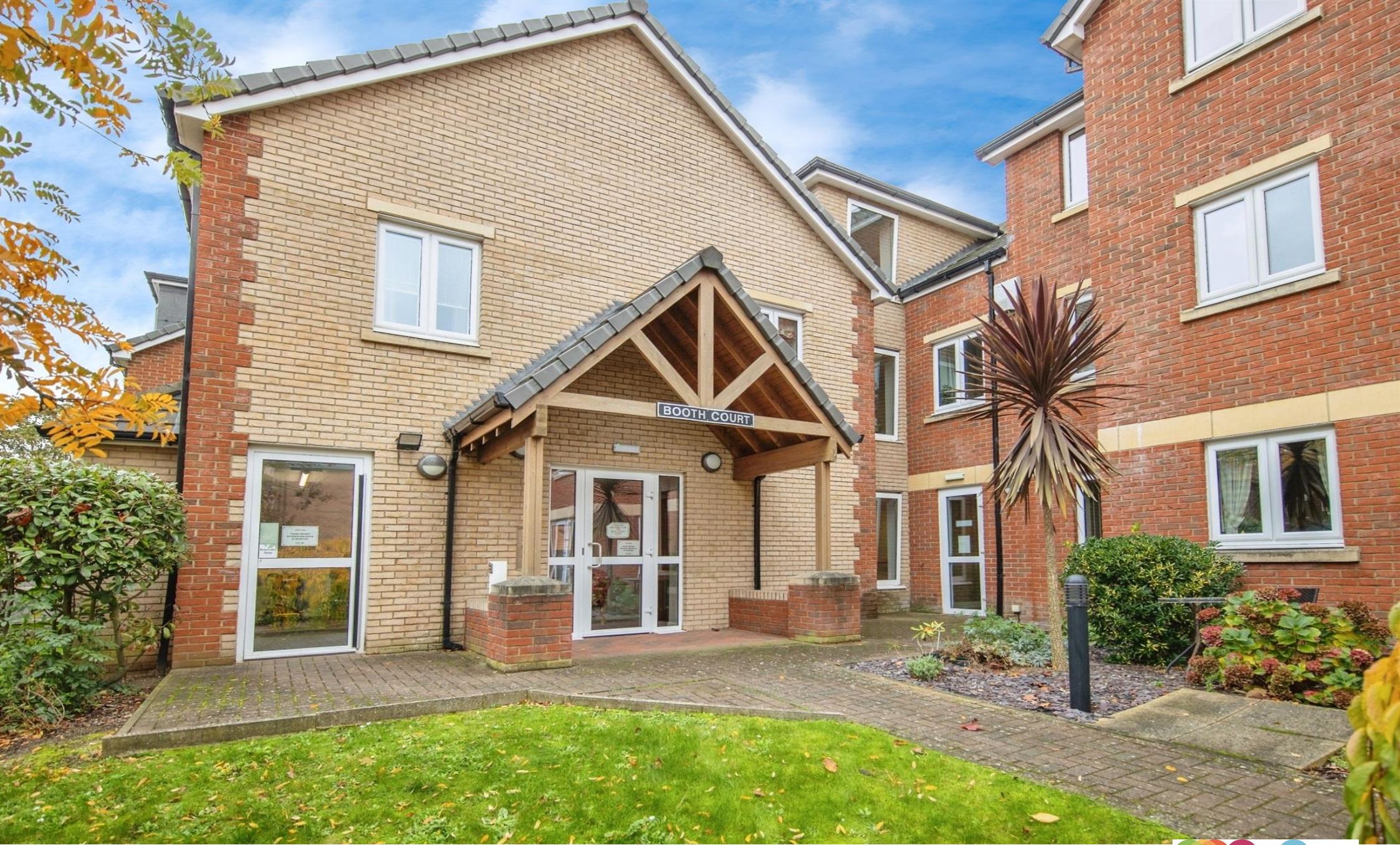
Booth Court, Handford Road, Ipswich, IP1 2GD
