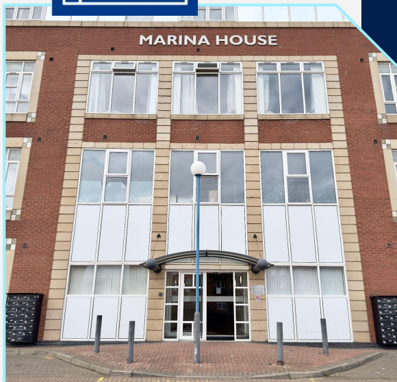
Marina House, Harbour Walk, Hartlepool, TS24
