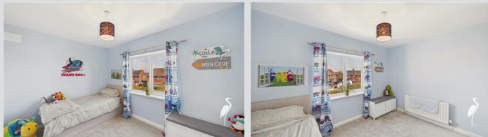
Double glazed window and radiator.
