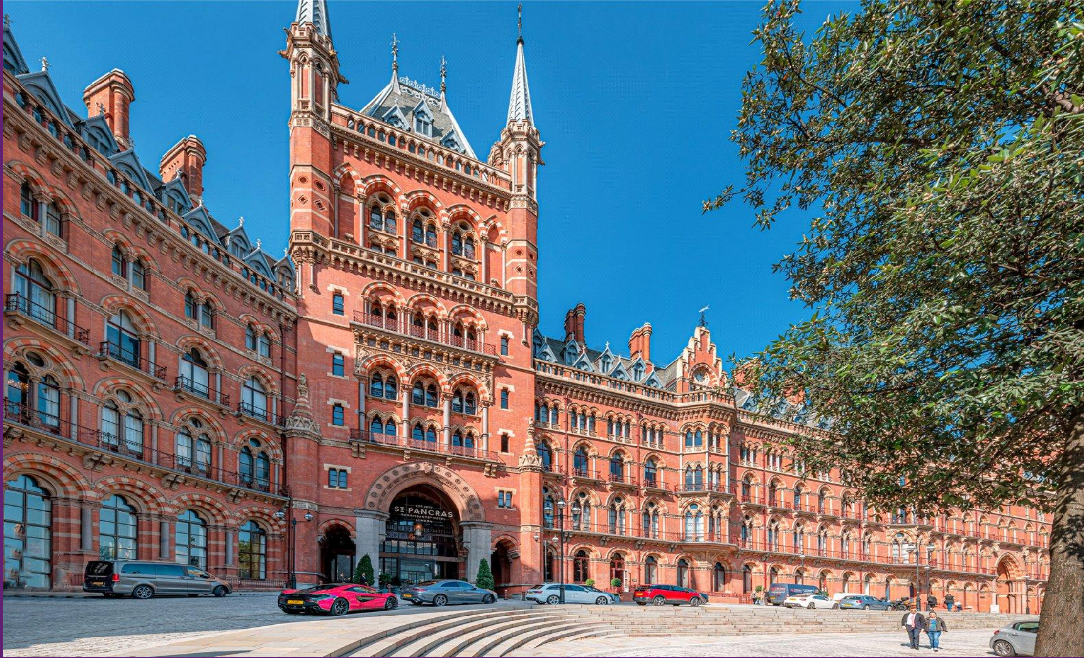
St. Pancras Chambers Euston Road, NW1
