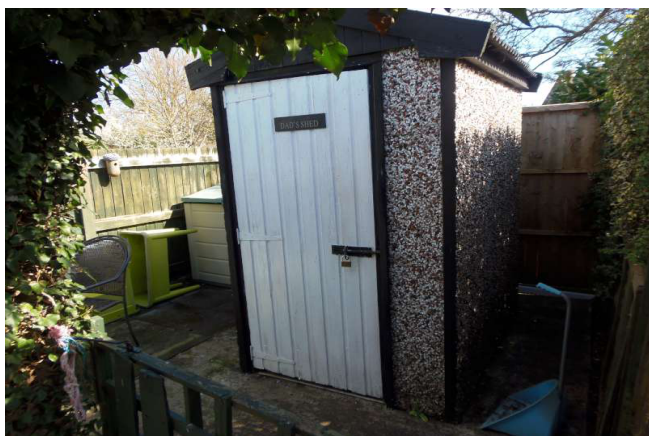
Gate to concealed store area with board fence, concealed frame store shed and store area.
