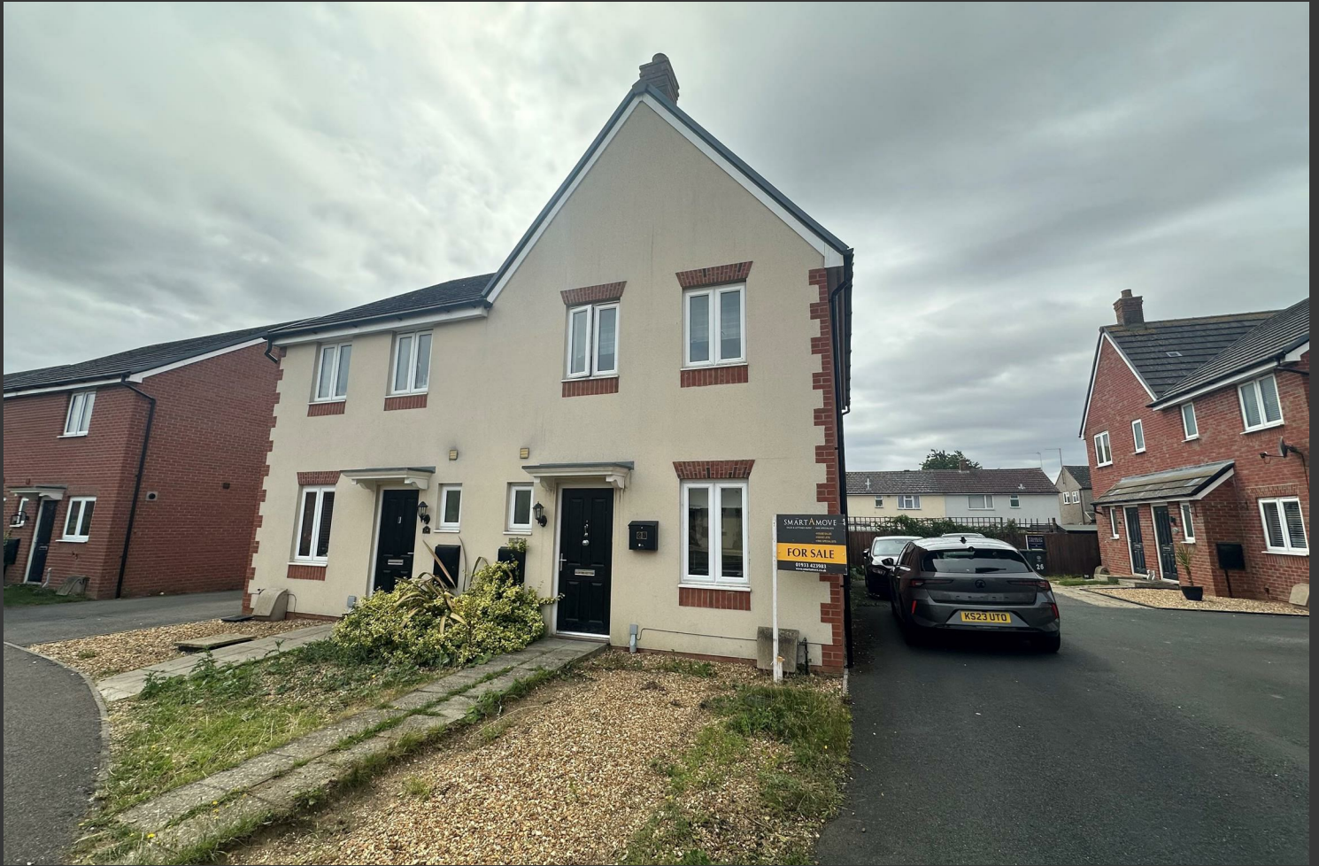
Chimney Crescent, Irthlingborough NN9 5WF
