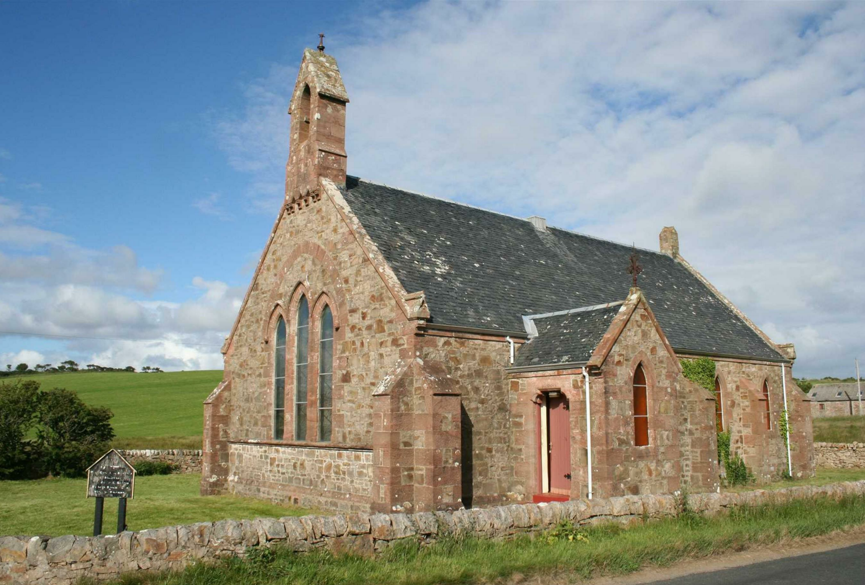
Bennecarrigan Church, The Ross Road, Sliddery, Isle of Arran, KA27 8PA
