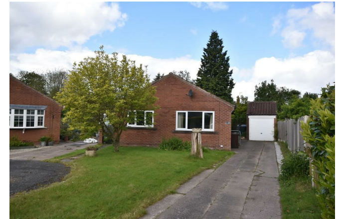
The bungalow is pleasantly situated in this quiet cul-de-sac location with views of the surrounding countryside. The spacious plot has a deep frontage, open plan front garden
