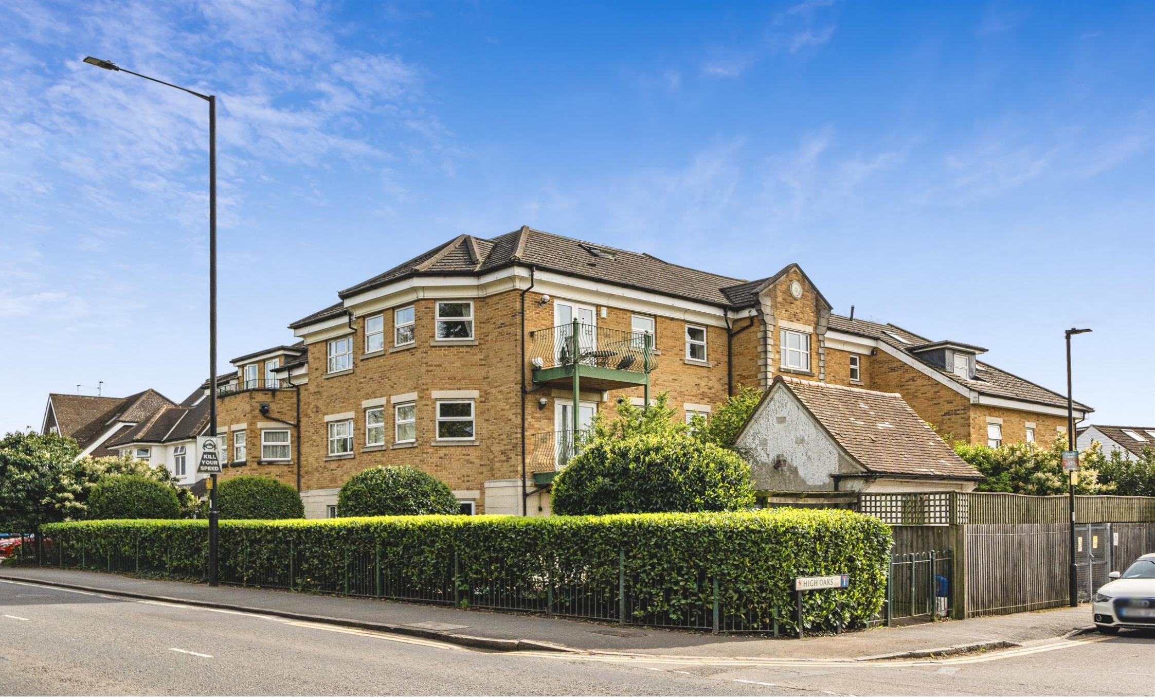
Holywell Lodge, The Ridgeway, Enfield, EN2 8JN
