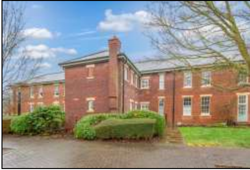
Side View of Building
