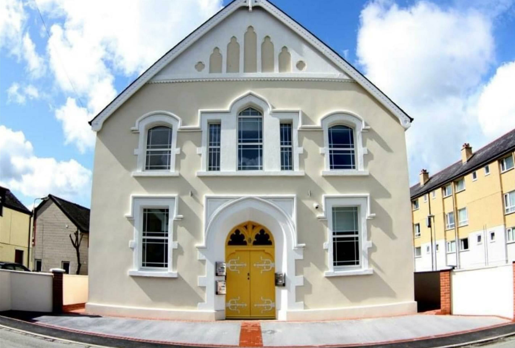
Seion Chapel Ambrose Street, Bangor 4 Bed House of Multiple
