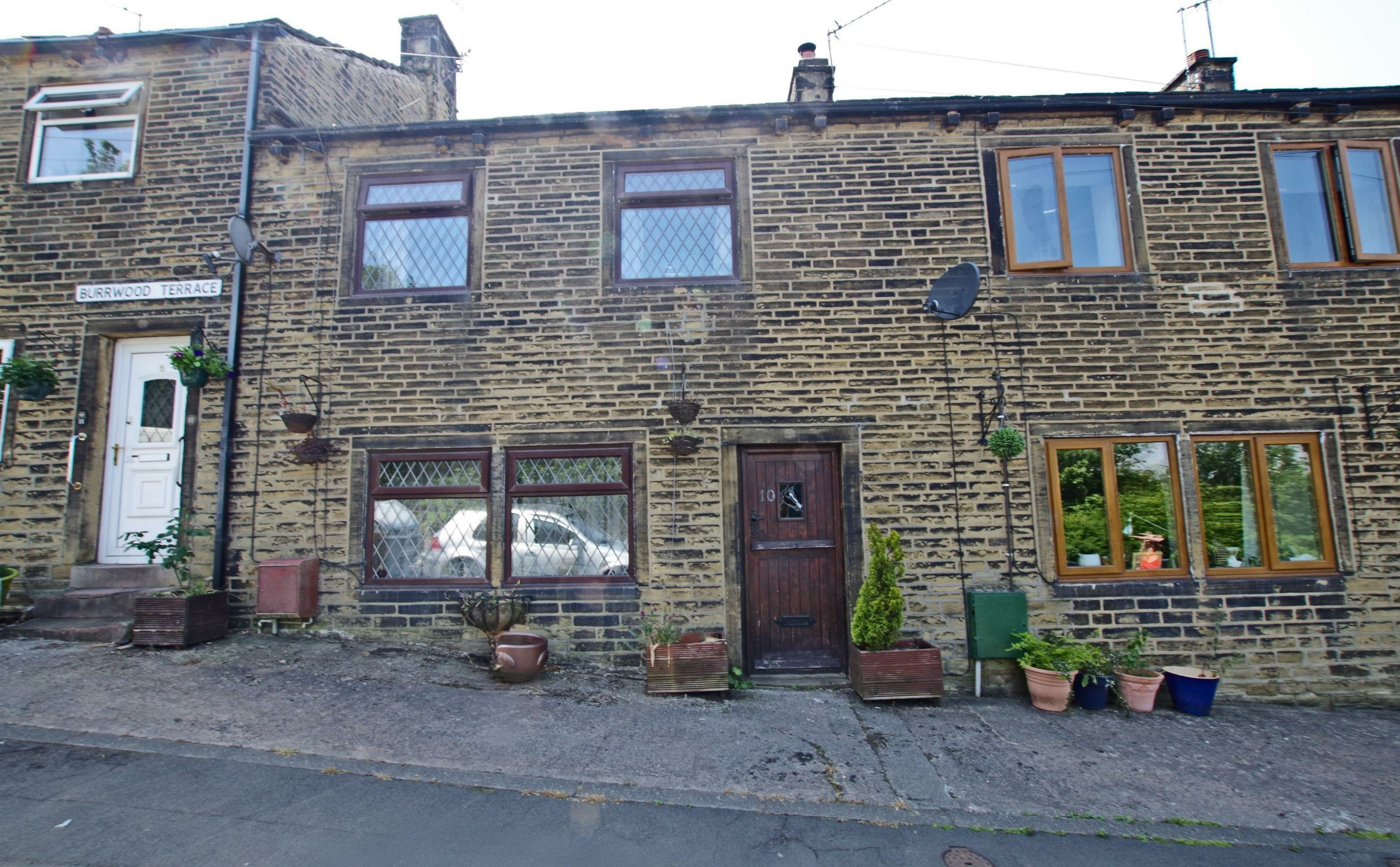
Burrwood Terrace, Holywell Green, HX4 9AL £190,000
