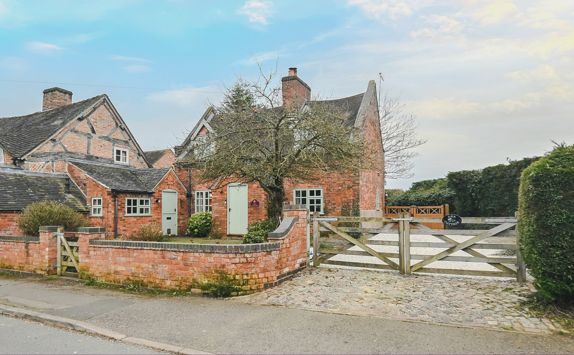
Lea Cottage, Hadley Street, Yoxall, DE13 8NB
