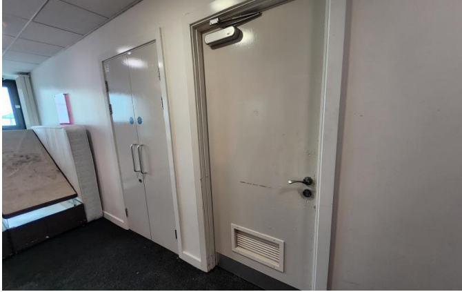
Maintenance manager's storeroom door.
