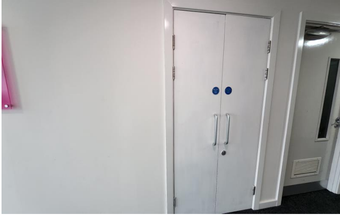
Example of a riser cupboard door.
