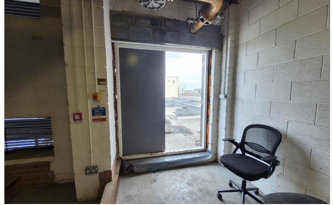
Roof access door.
