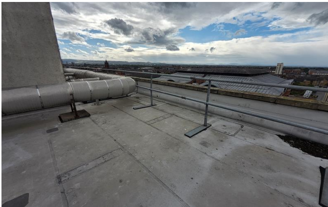
Barriers on the roof.
