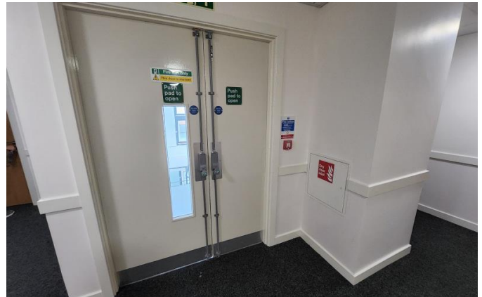
'Push pad to open' fire exit signs.
