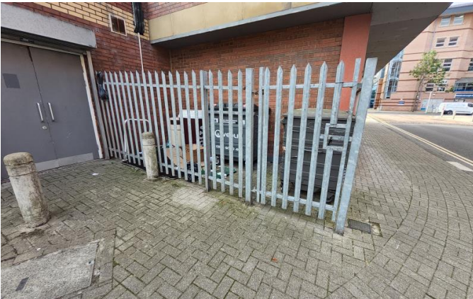
External bin storage area to the rear of the building.
