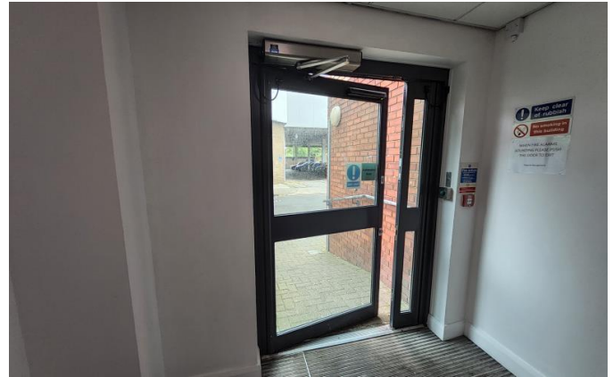
Rear fire exit door.
