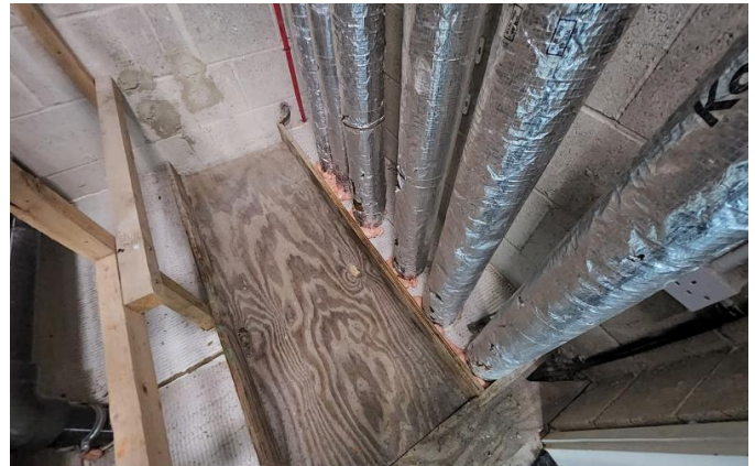
Expanding foam used to fire-stop gaps in the riser cupboards.
