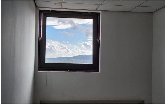
Example of an openable window in the protected stair core.
