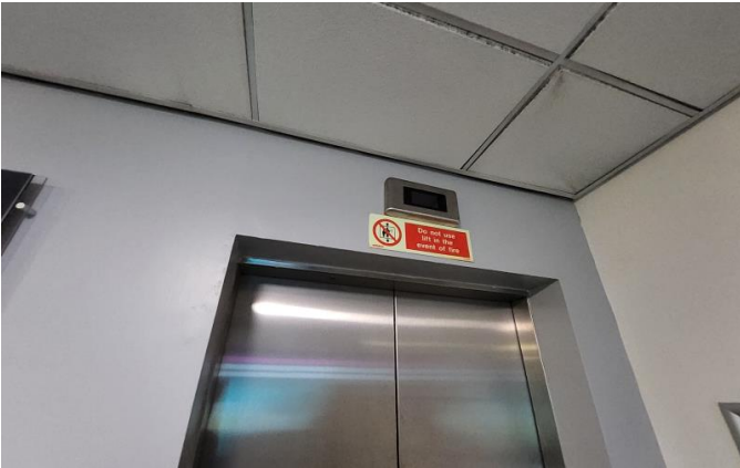
Example of a lift warning sign on the ground floor lifts.
