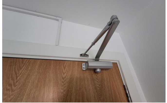
Room 6-01's front entrance door's positive self-closing device.
