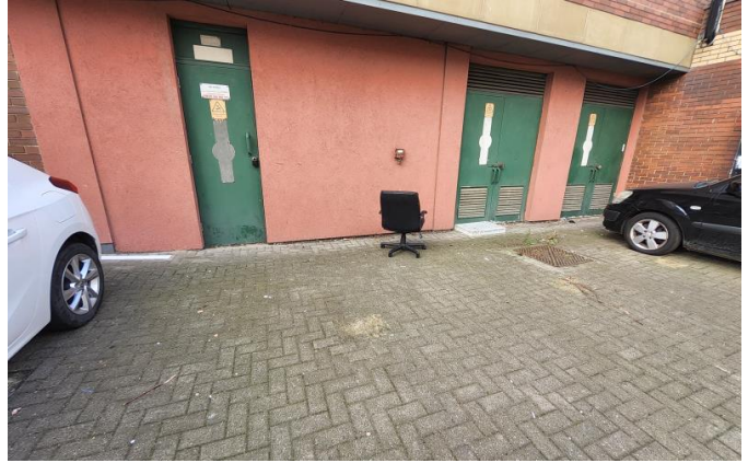
Office furniture to the rear of the building.
