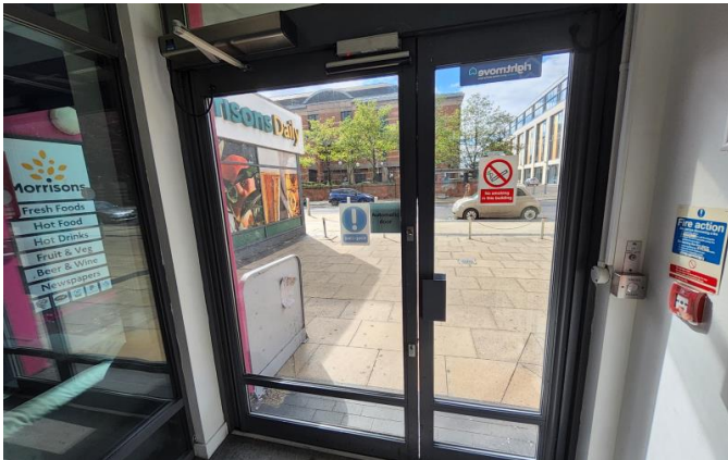
Glazing systems are marked.
