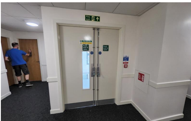
Fire exit directional signs visible.
