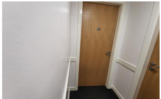
Room 2-39's front entrance door.
