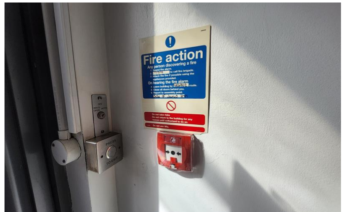
Front entrance/exit door.
