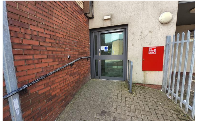
External emergency lighting.
