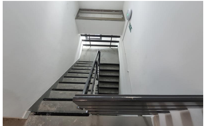
Protected stair core.
