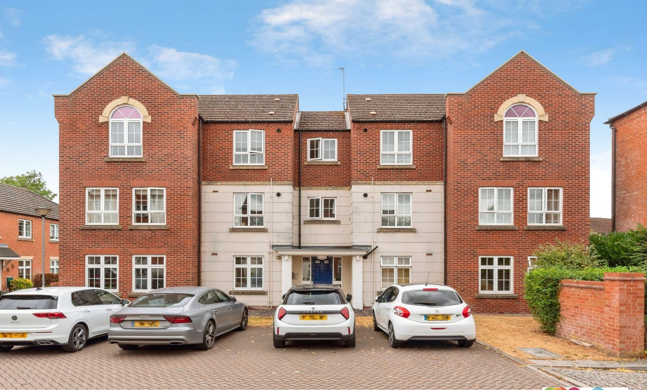
Palmers Court, Southwell NG25 0JG
