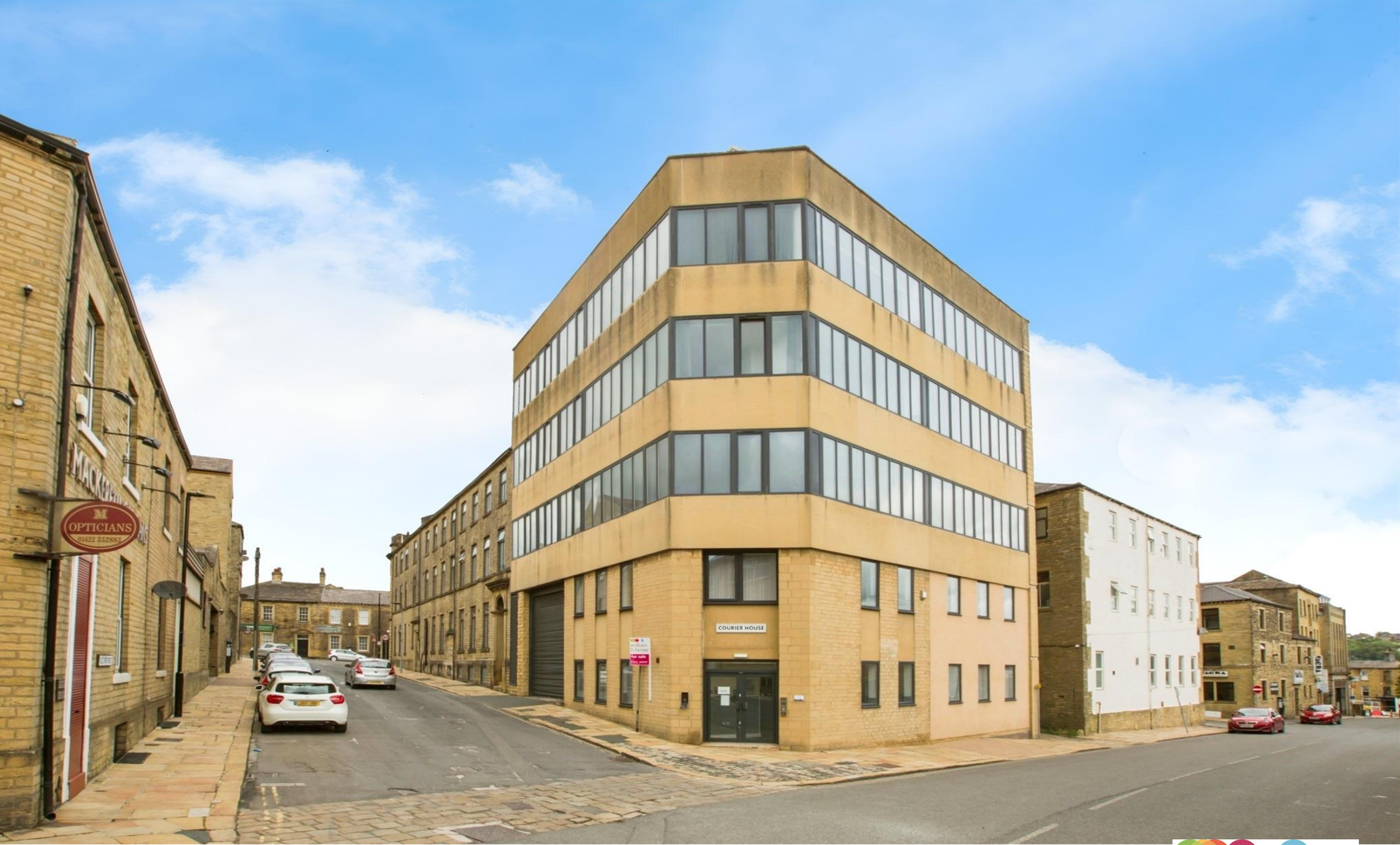
Courier House, King Cross Street, Halifax, HX1 2DG
