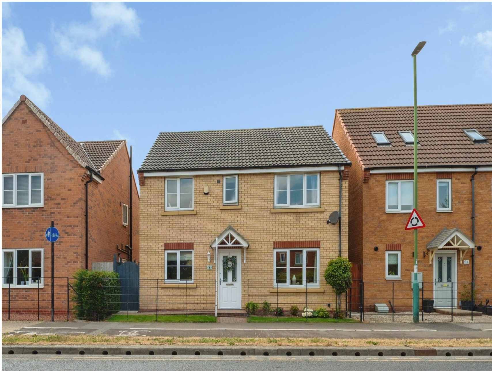
Richmond Lane, Kingswood, Hull, HU7 3AE
