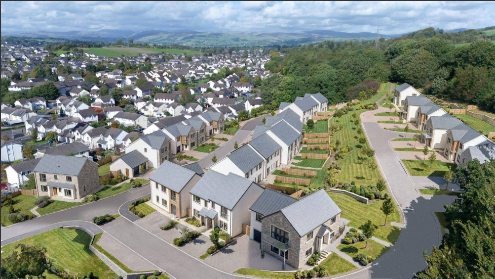
FROM THE SITE, LOOKING NORTH-WEST OVER KENDAL TOWARDS THE LAKELAND FELS
