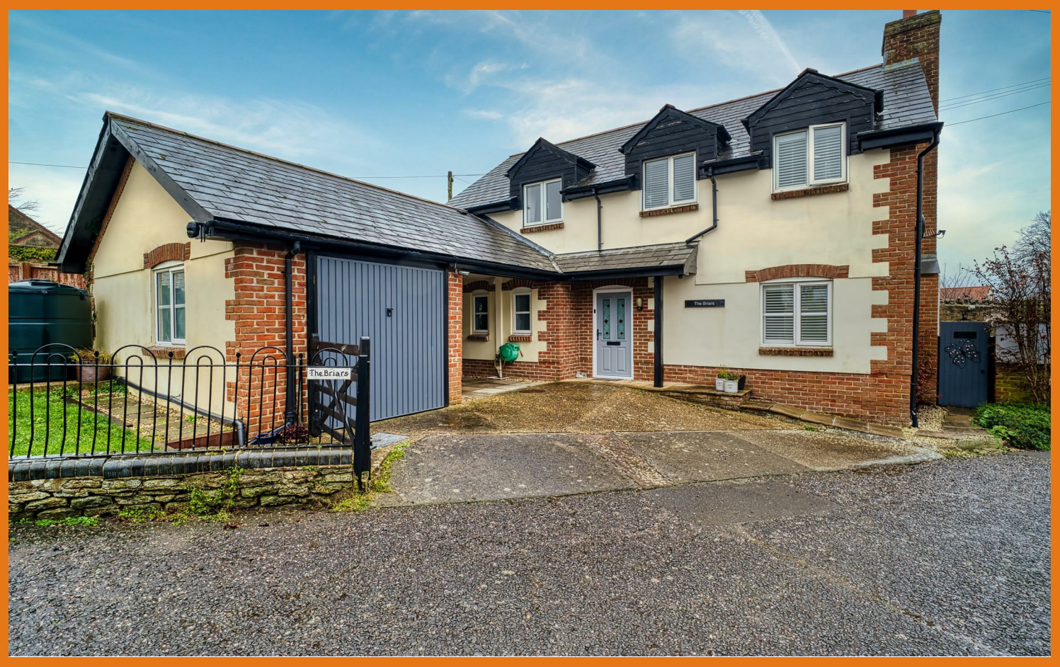
Church Hill Templecombe
