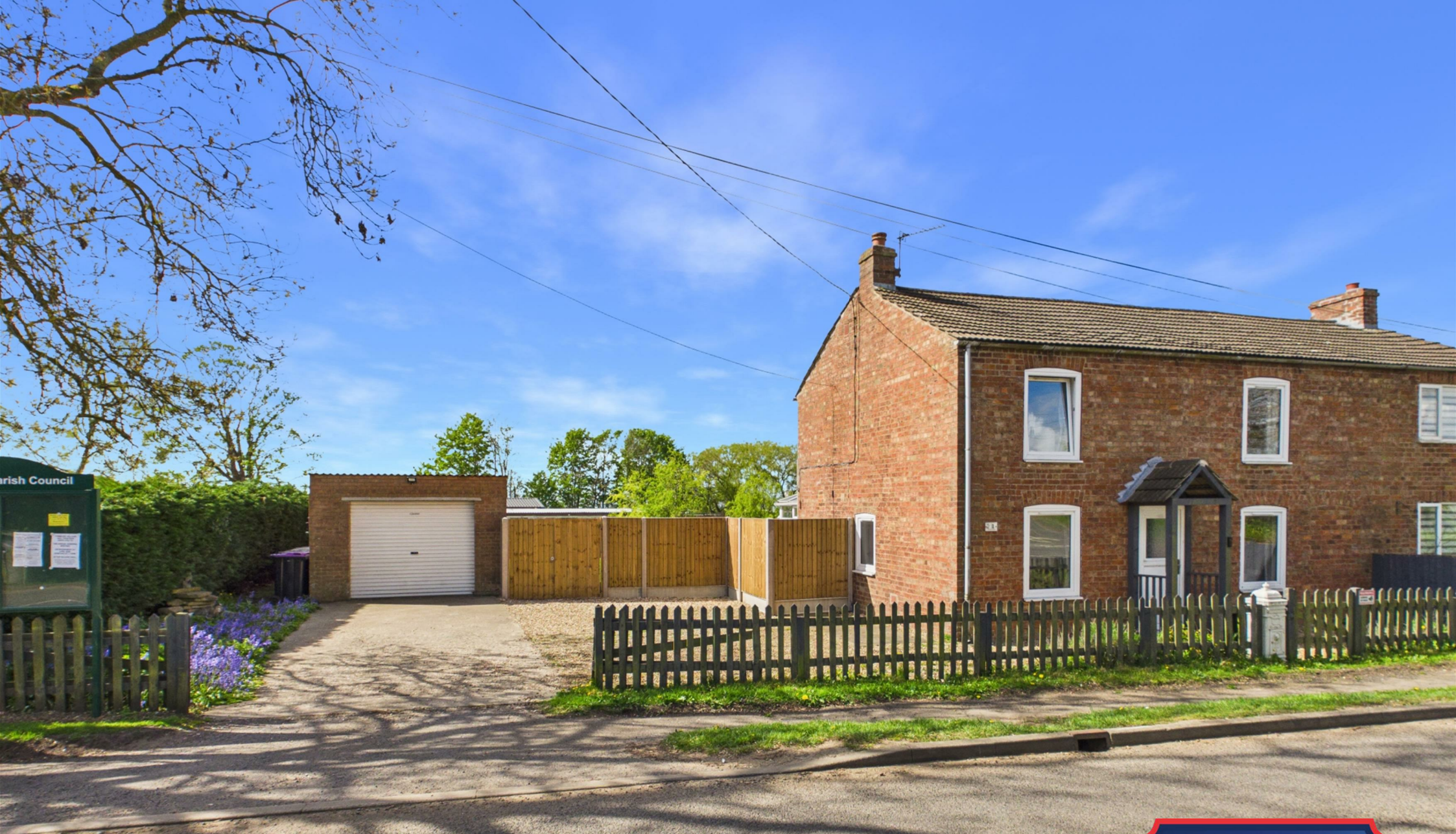
I Cleveleys Cottage, Main Road Thimbleby, Horncastle, Lincolnshire, LN9 5RB
