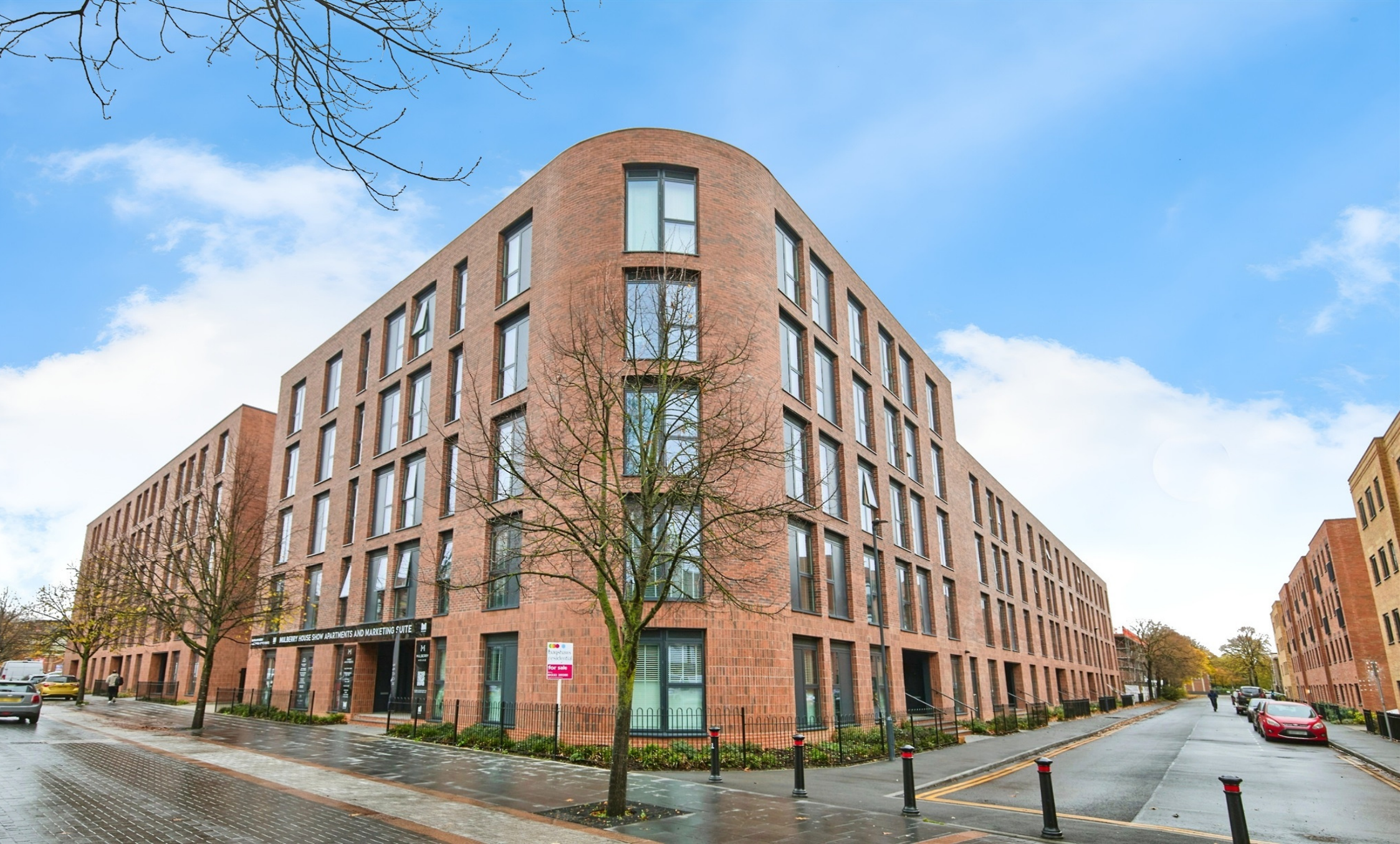
Mulberry House Castleward Boulevard, Derby DE1 2FQ
