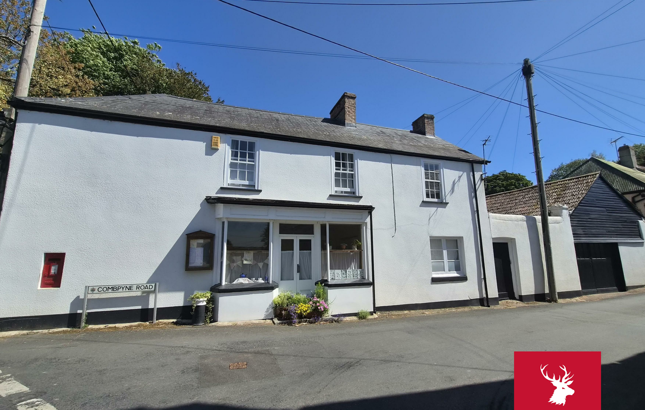
The Post House, Church Hill
