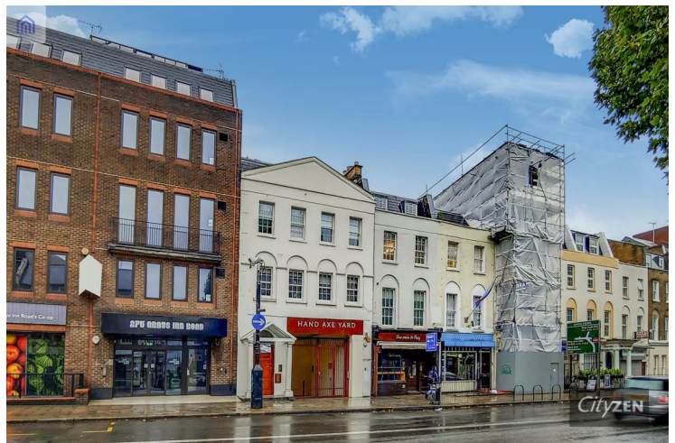
GATED ENTRANCE FROM GRAYS INN RD
