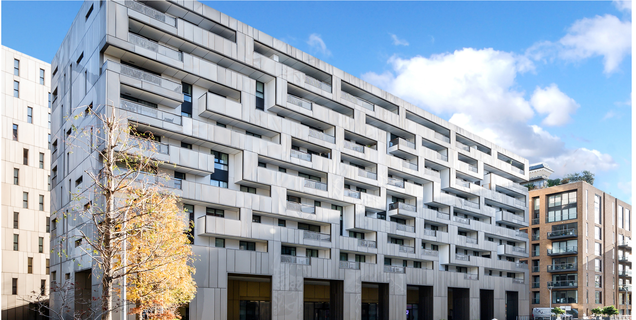
BRAMAH HOUSE, Battersea SW1W
