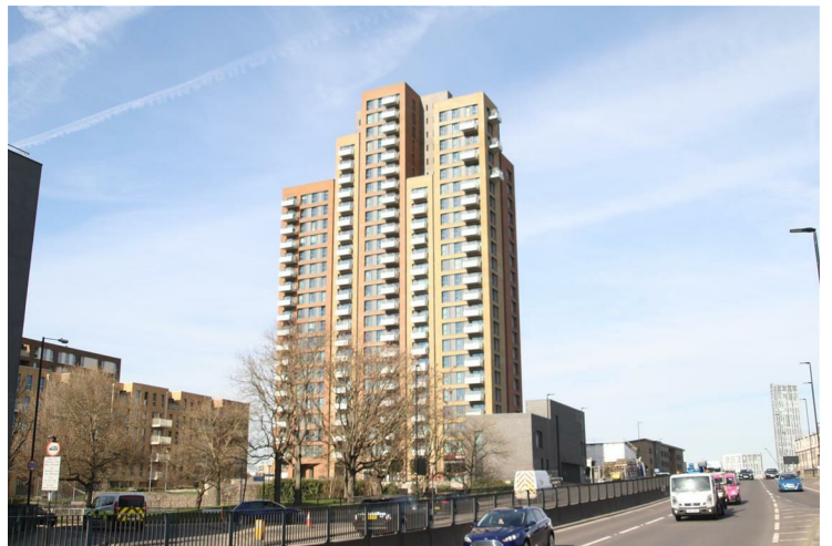
MARNER POINT BUILDING
