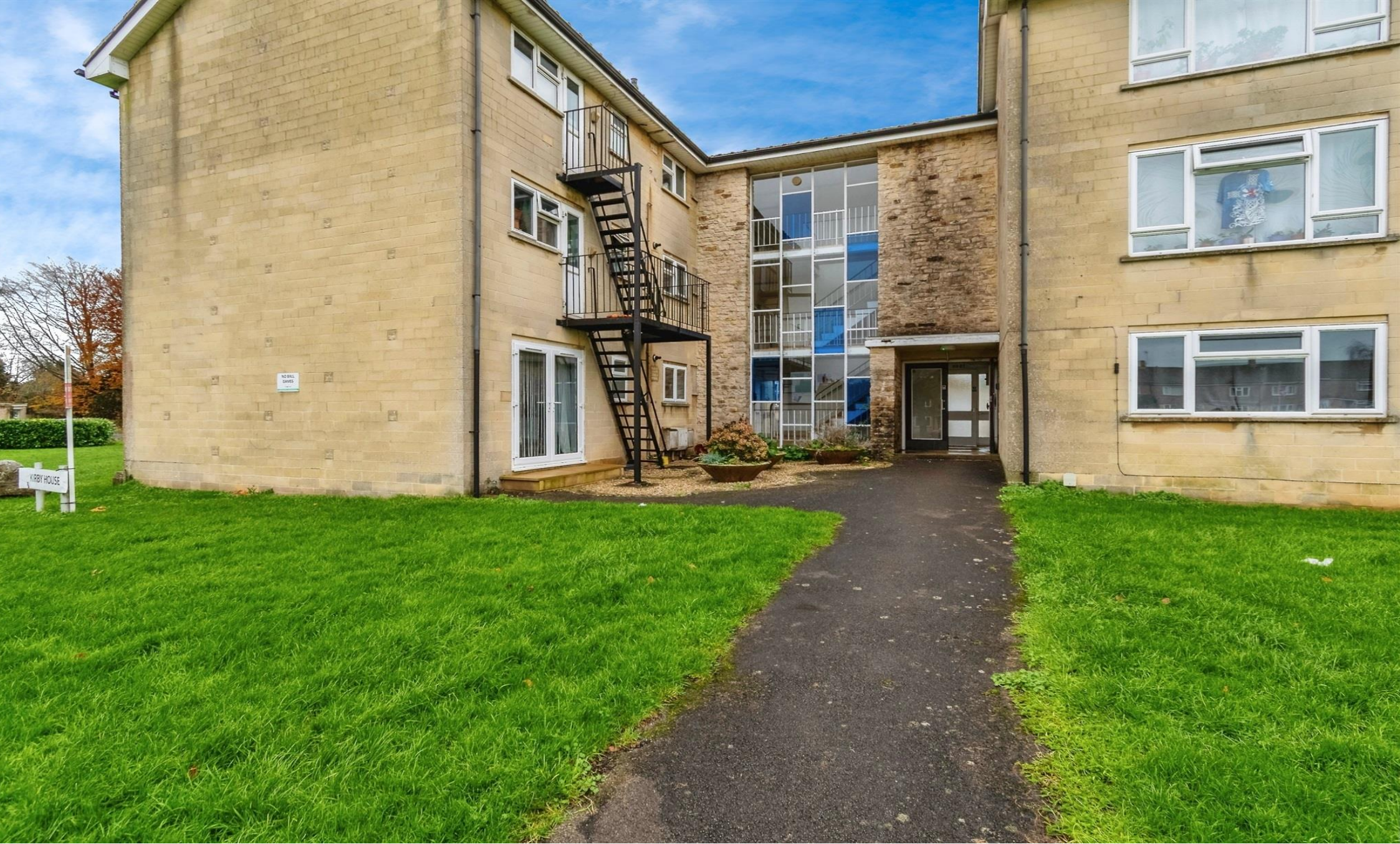
Kirby House, Methuen Way Corsham SN13 0EJ
