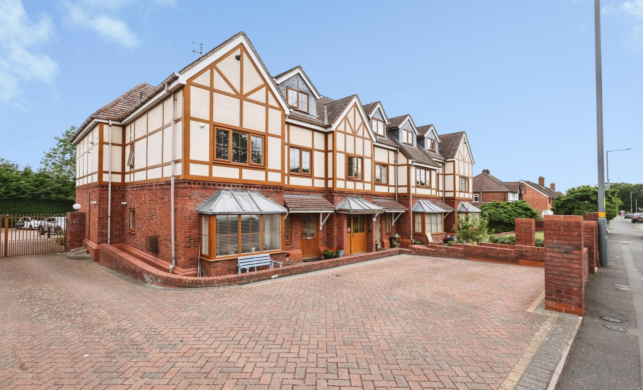
Barrows Manor, Barrows Lane, Birmingham
