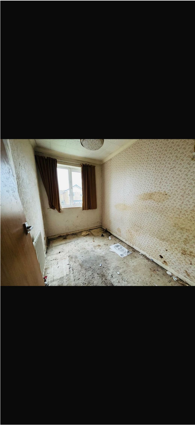
Double glazed window, central heating radiator
