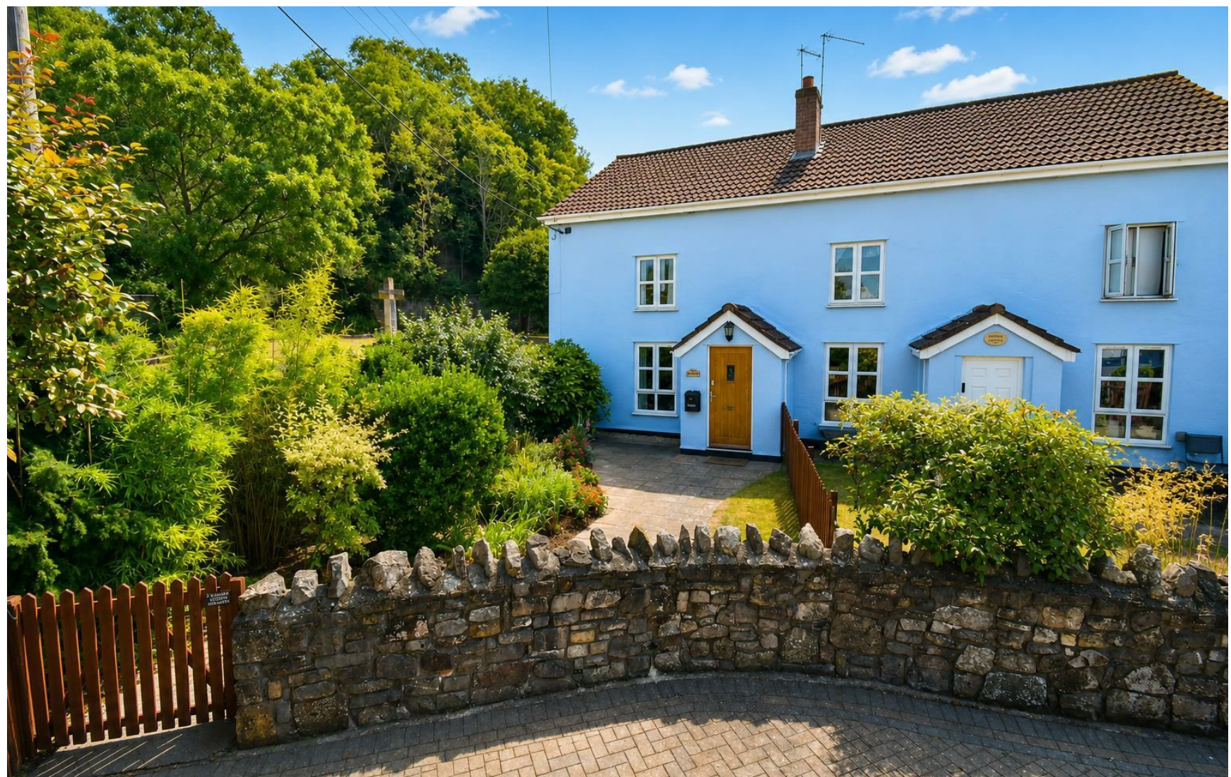
MARSH COTTAGE MOORHOUSE LANE
