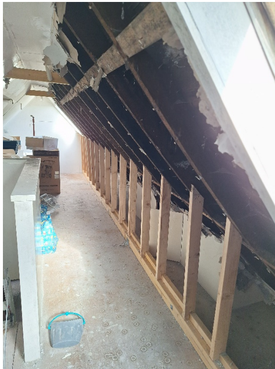
Photograph 4 – Existing attic space with temporary roof propping
