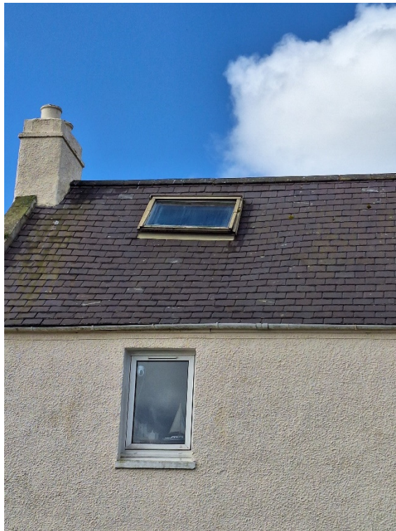
Photograph 2 – Sagging to the roof around the rooflights
