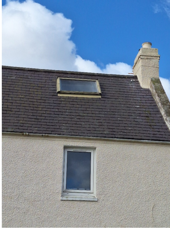
Photograph 2 – Sagging to the roof around the rooflights
