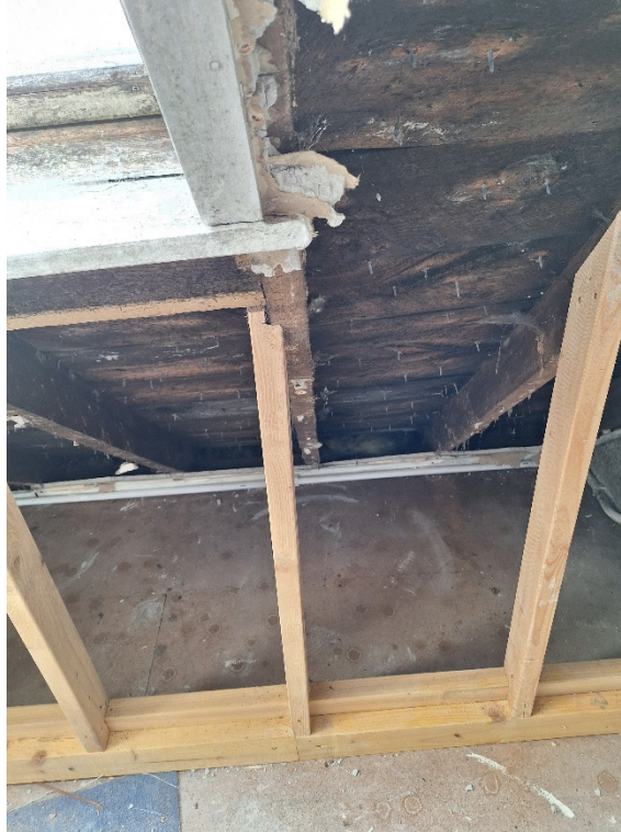
Photograph 5 – Roof light trimmers
