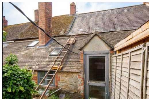
Rear Roof in slate
