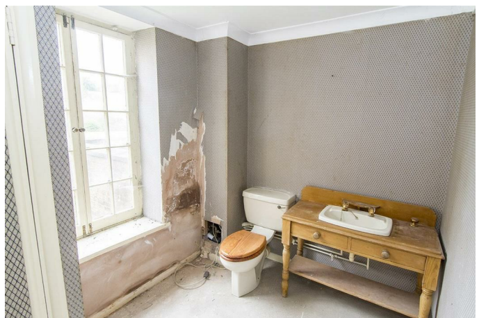
Ground Floor Bathroom 9'8 x 6'10 (2.95m x 2.08m)
