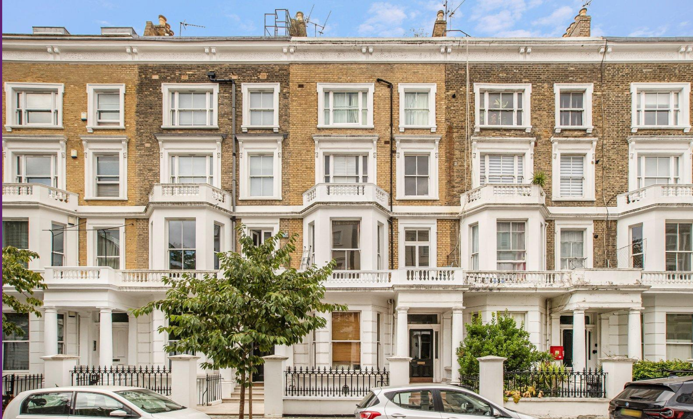
Lexham Gardens Kensington, W8
