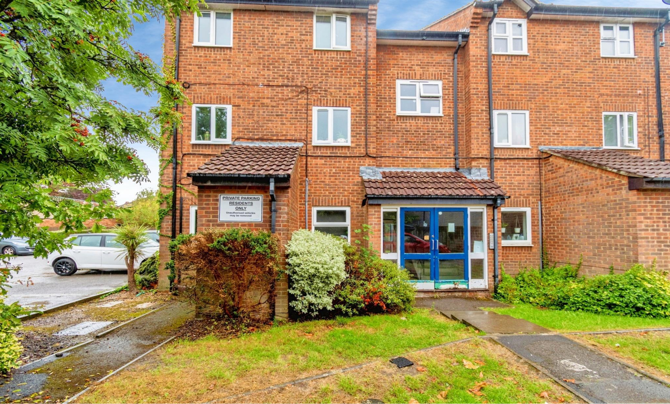
Kingsmead Court, Yarmouth Gardens, SOUTHAMPTON SO15 5SF
