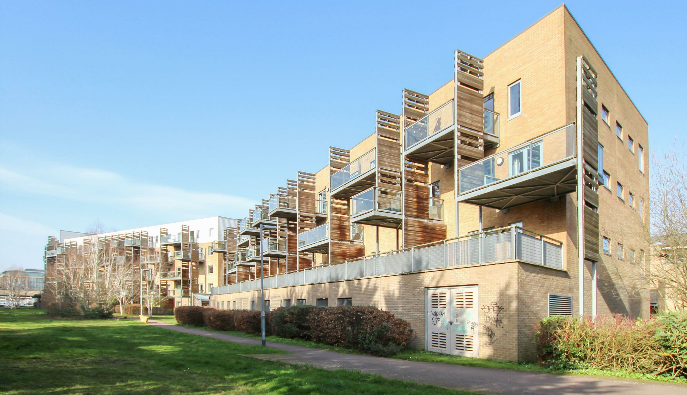
Bailey House, Rustat Avenue, Cambridge, CB1 3PG
