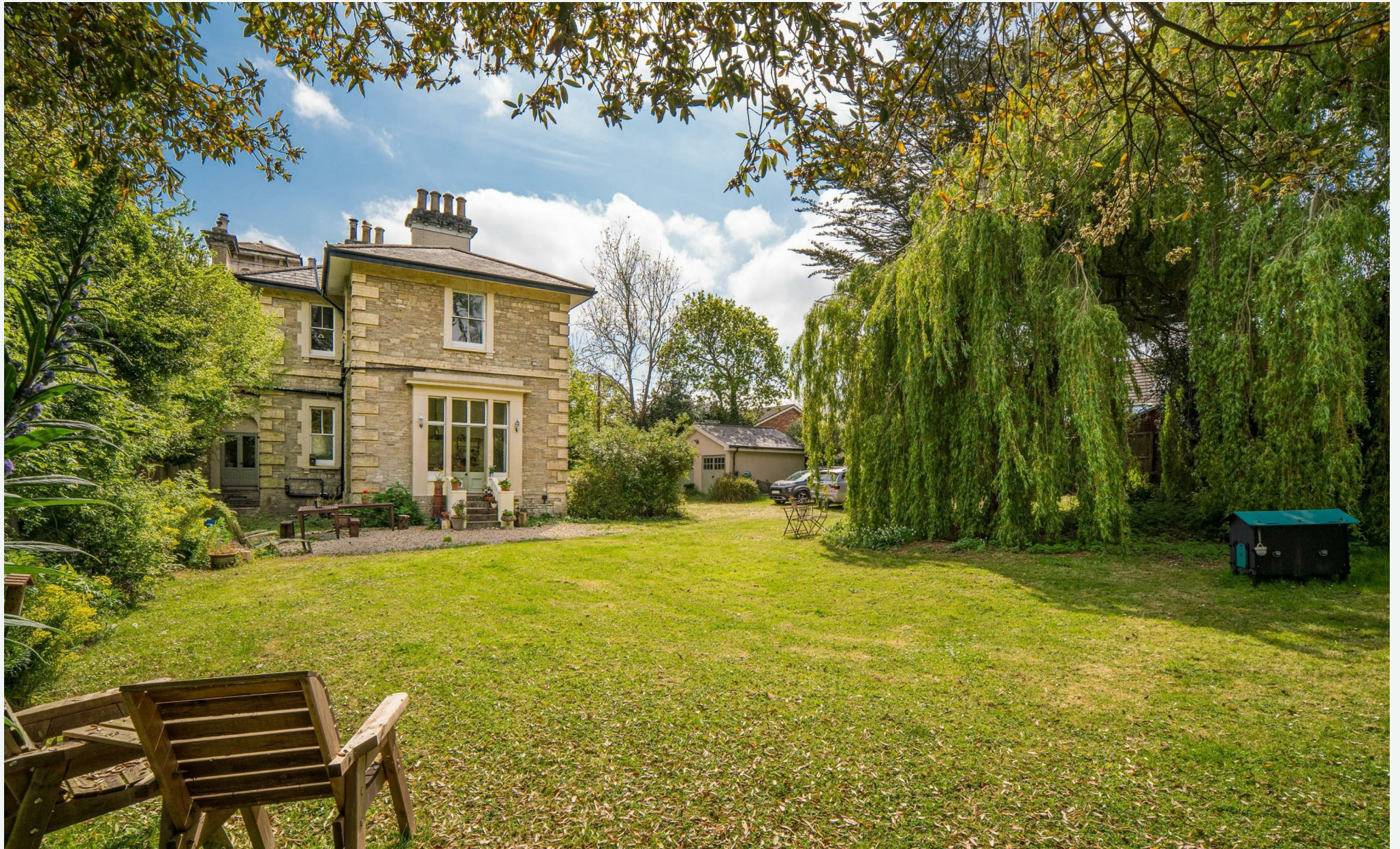
Willow House, Church Road, Binstead, Isle Of Wight, PO33 3TB
