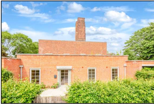
Elevated Front View
