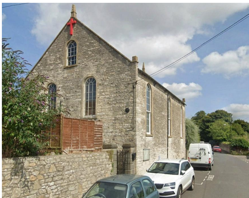
Fig. 2 – photograph of South Road Methodist Church from west side
