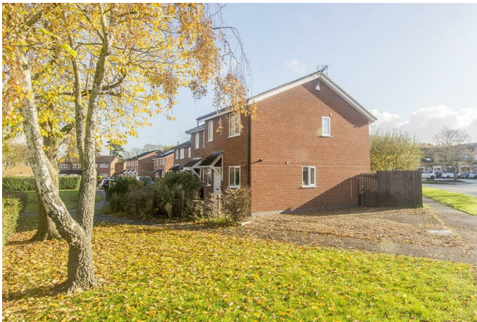
Side Elevation photo
