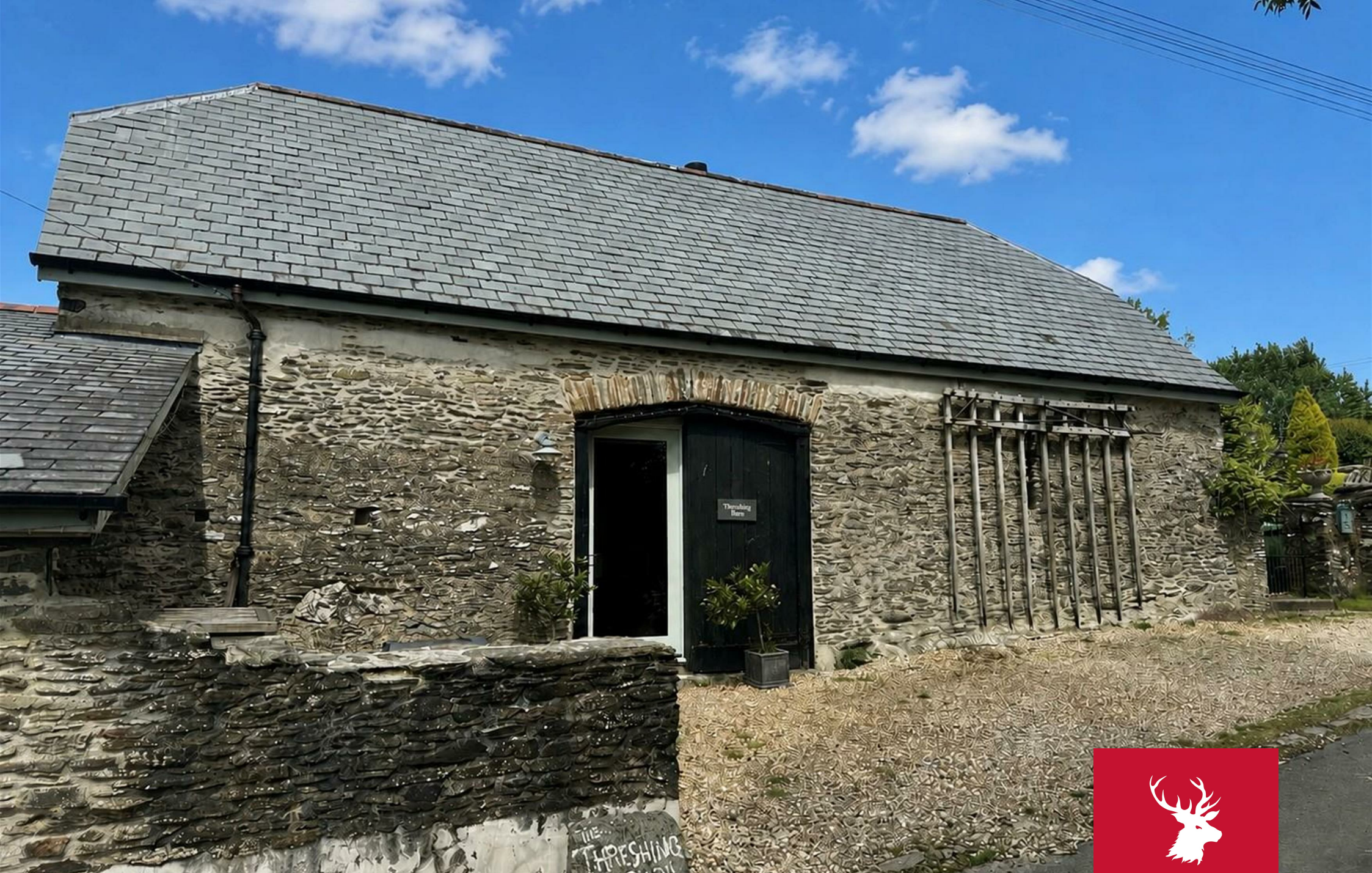
The Threshing Barn
