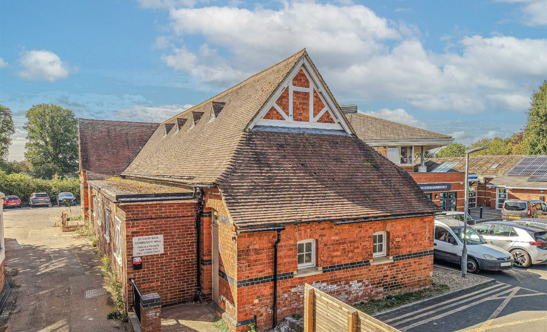
Parish Church Hall, Coventry Road Market Harborough, Leicestershire, LE16 9BX
