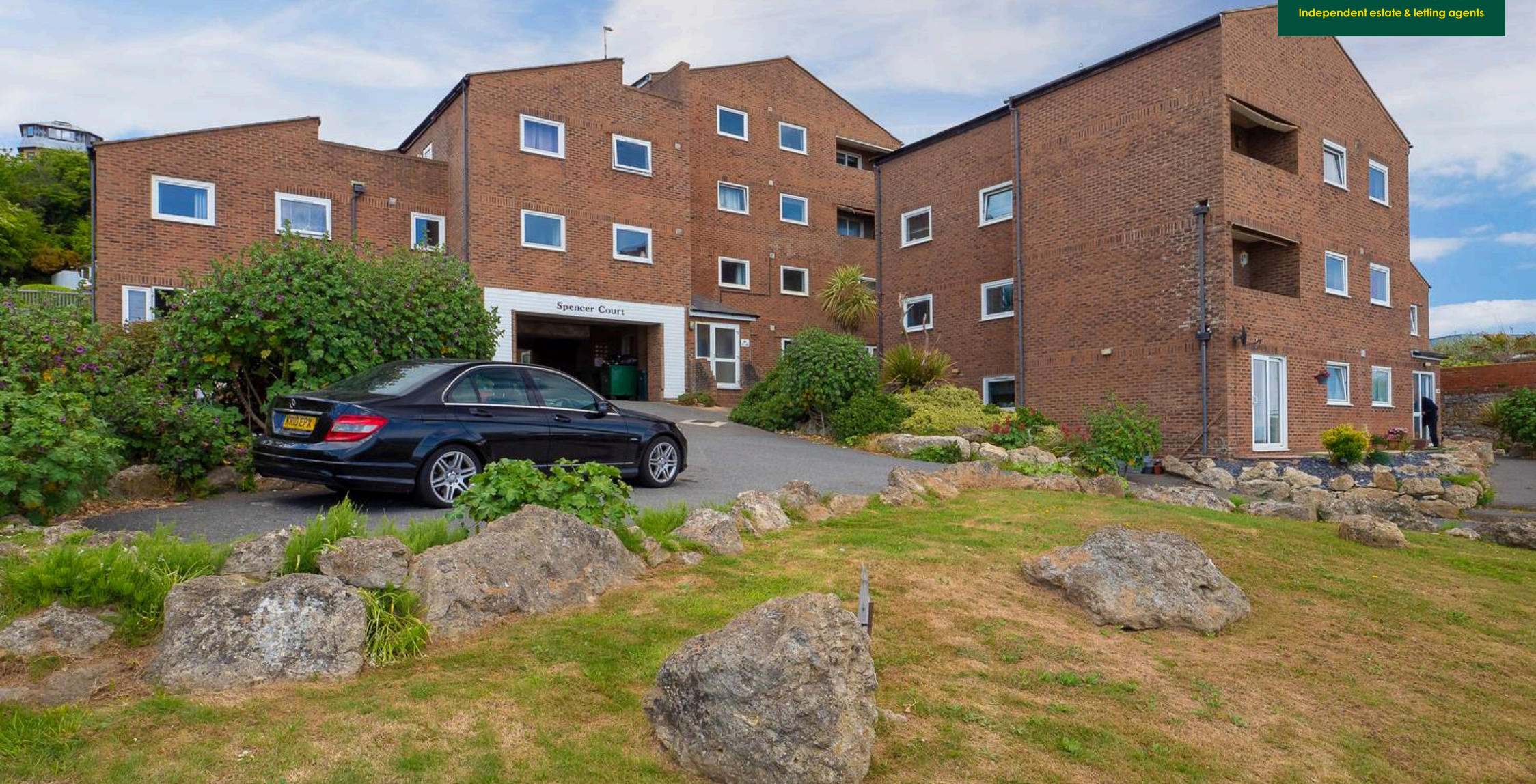
25 Spencer Court Sandgate Esplanade, Sandgate - CT20 3TJ £850 pcm
