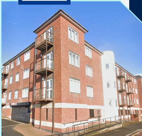
Toll Bar House, Ryhope Road, Sunderland, SR2
