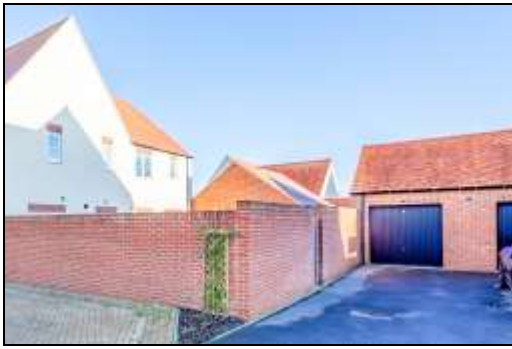
Garage with electric door
