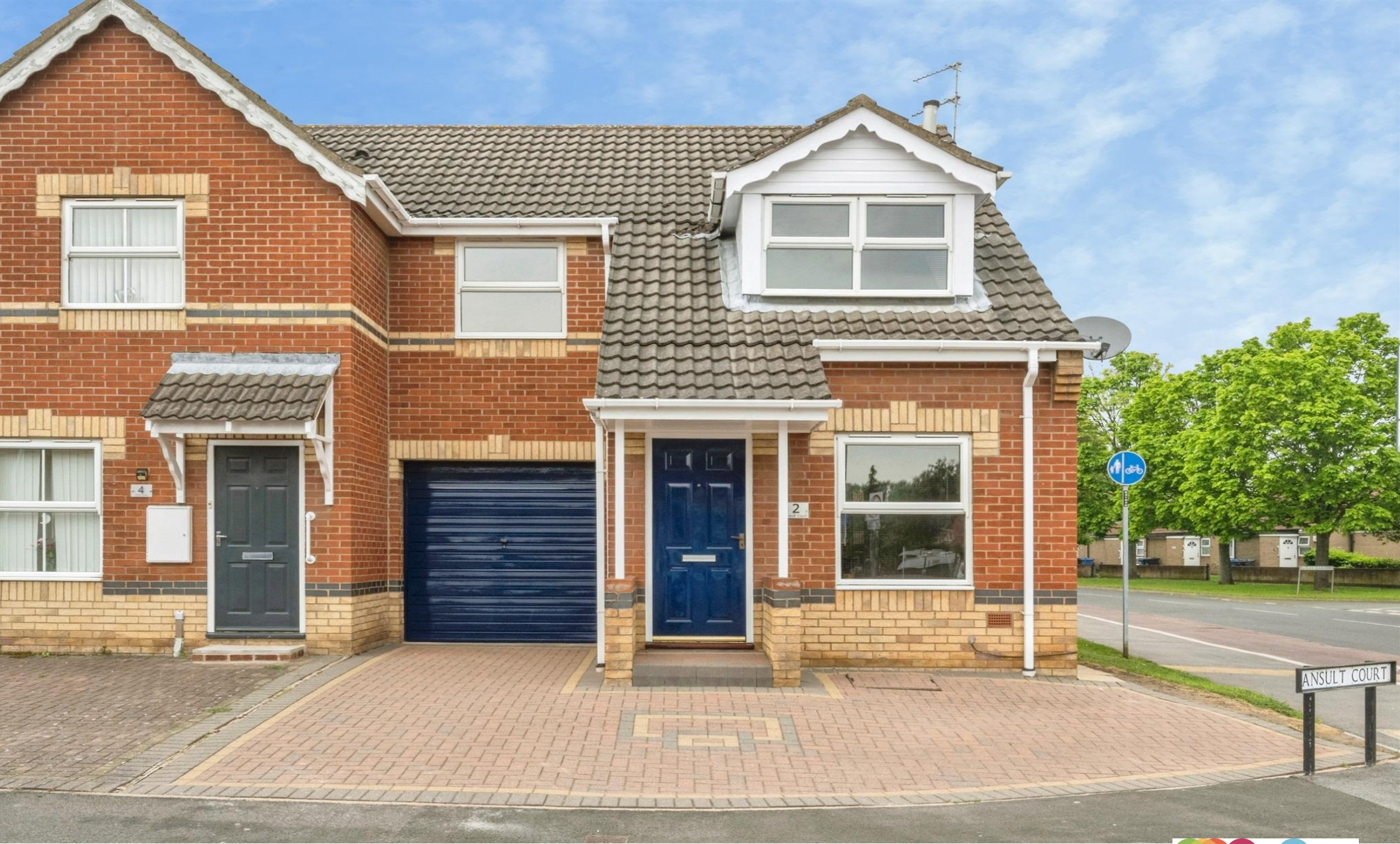
Ansult Court, Bentley Doncaster
