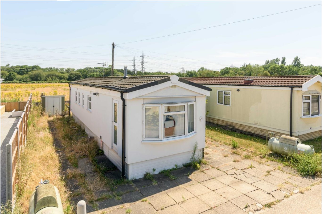
19 Avenue C Weybridge Park Estate Addlestone Surrey KT15 2RB
