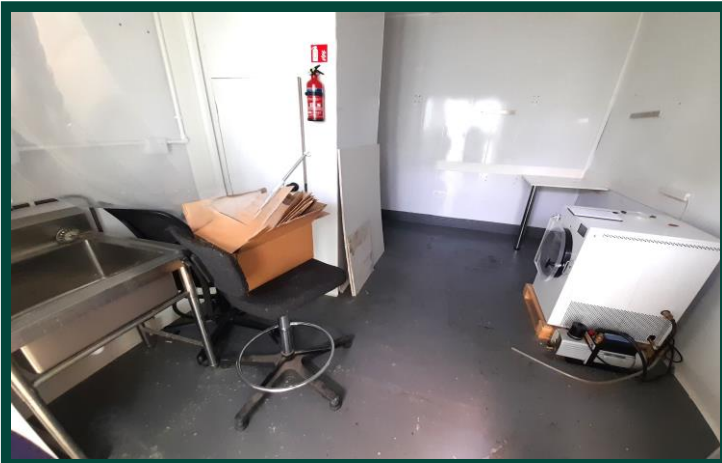
Ground Floor – Food Prep Room
