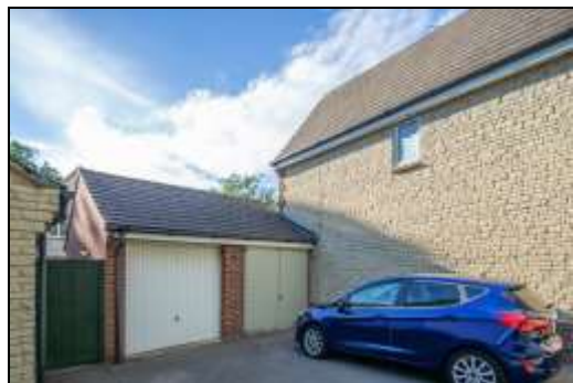
Garage and Driveway Parking
